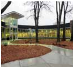
Clayton County Forest Park Branch Library Hogan Construction Group
