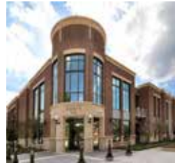
Augusta-Richmond County Sheriff's Office Heery International Potts Construction
