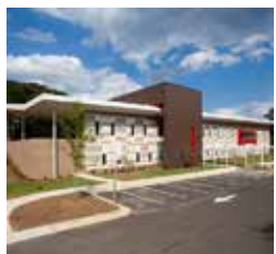
Adamsville Regional Health Center The Whiting-Turner Contracting Company
