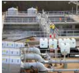
Piedmont Regional Wastewater Treatment Plant MWH Constructors
